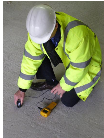
Concrete temperature +5°C and rising
