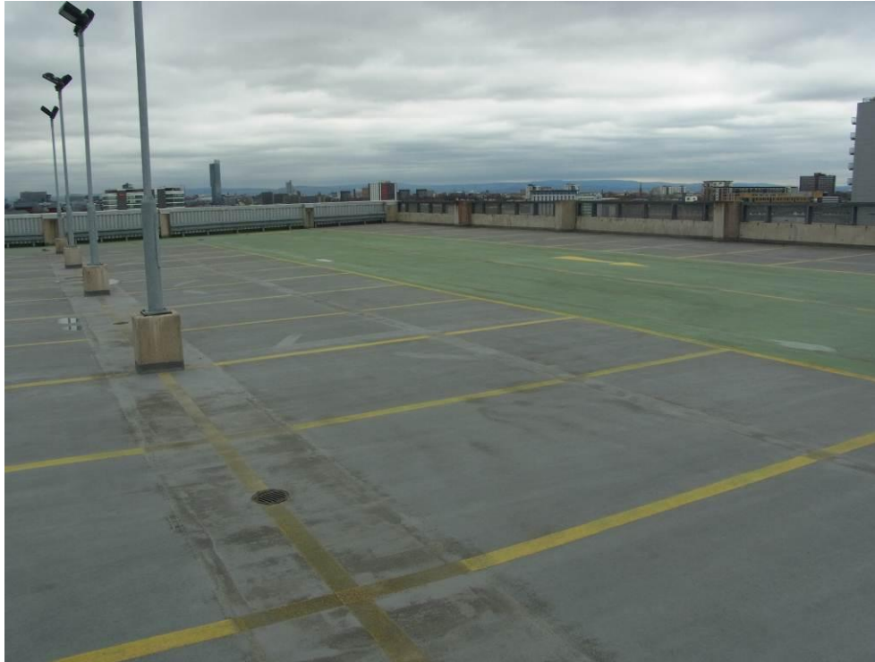
Figure 3 General view of Lowry Centre car park
