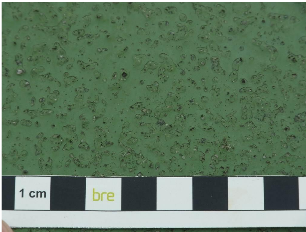
Figure 4 Lowry Centre, localised abrasion of pigmented top coat
